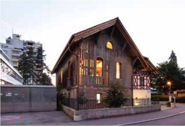
Office and residential building Julia Kick, Julia Kick (2017)
